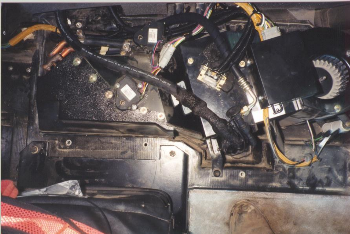
Evaporator box reassembled with hoses, and preset thermostat in place
