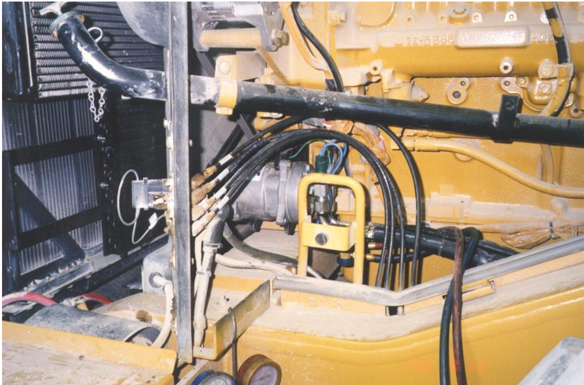
Compressor in place on mount with rotolocks, binary switch and hoses.
